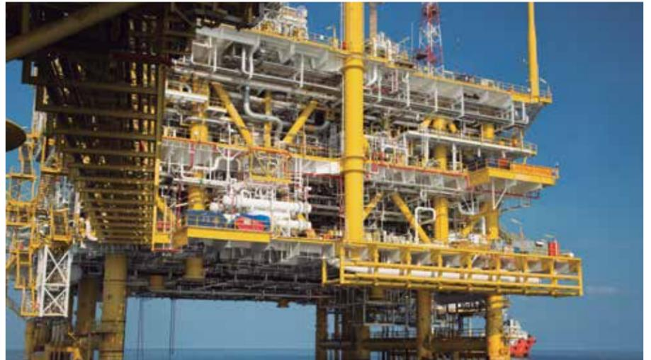
Many oil platforms located in the North Sea are constructed of stainless hollow sections manufactured by Stalutube.
